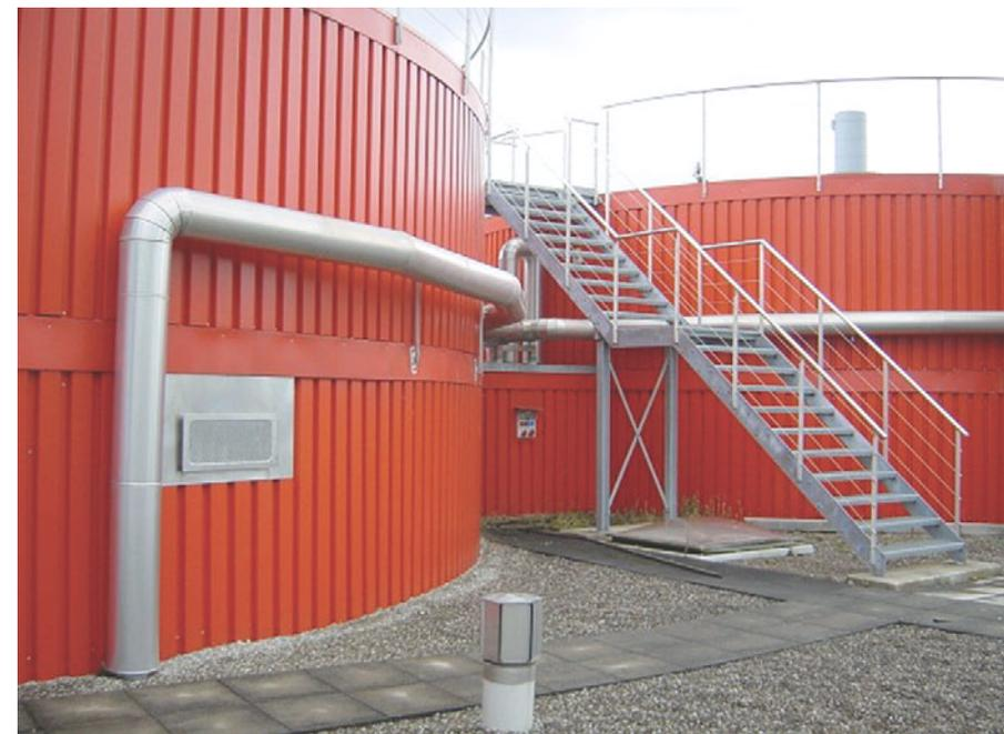
Figure 16: Two fermentation tanks with integrated gasometers<sup>1)</sup>
