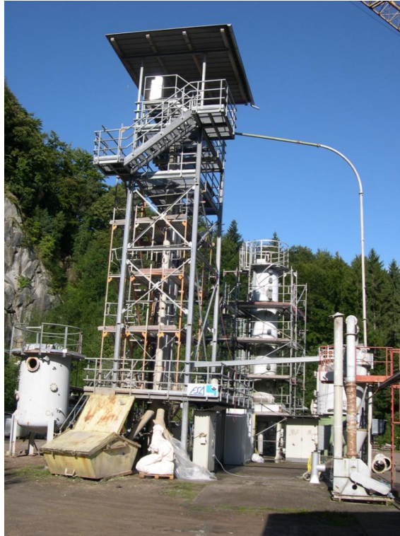
Figure A1: The test elevator surrounded by scaffolding, on the right the dedusting pipe
